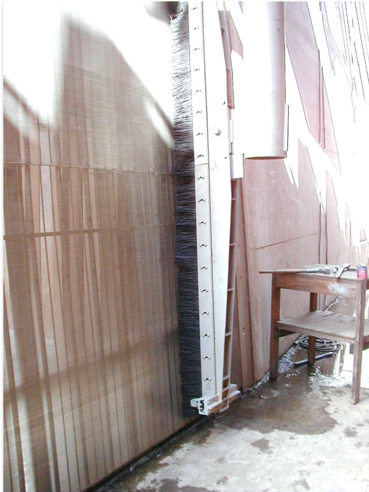
Figure 2. Picture of a flat-plate screen wiper blade. Entire structure dewatered during construction. Picture by Dave Vogel.
