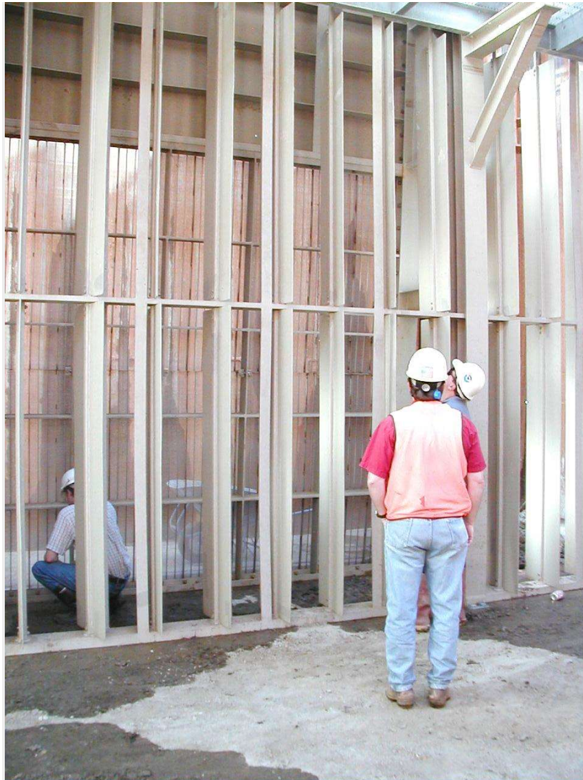
Figure 1. Picture of flow-control baffles in the open position (foreground) and flat-plate screens in the background. Entire structure dewatered during construction. Picture by Dave Vogel.
